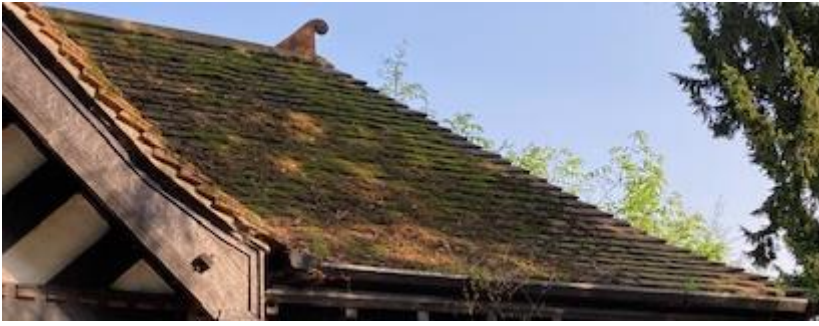
Appendix D – Guttering on Rockley Park Pavilion
