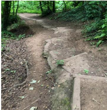
Appendix C – Missing handrail and uneven ground
