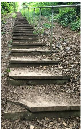
Appendix B – Missing handrail and poorly maintained steps
